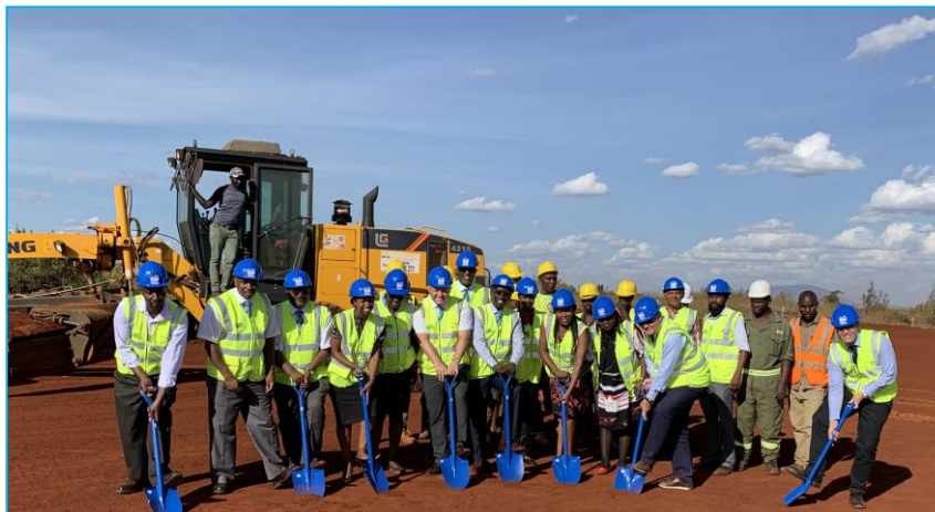
Chairman Alec Davis, CEO David Gatende, other Executives and some of the Supply team staff together with representatives of contractor Ark Construction celebrate ground-breaking for the new D&S Distribution Centre at Tatu City.
