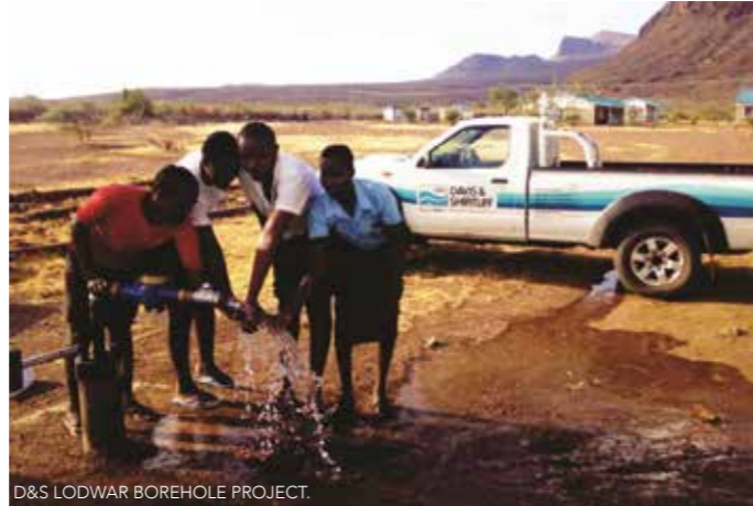
D&S LODWAR BOREHOLE PROJECT.
