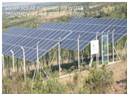
66KWP SOLAR POWERED RO WATER TREATMENT PLANT IN LAMU, KENYA
